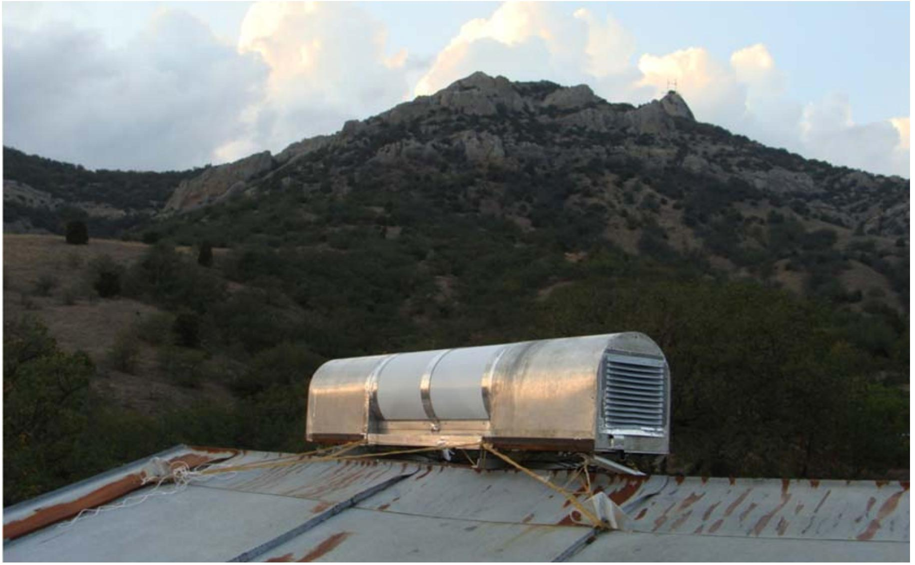
2020-2021 The device is without insulation. View from the facade. Air passes through the side ventilation grilles.
